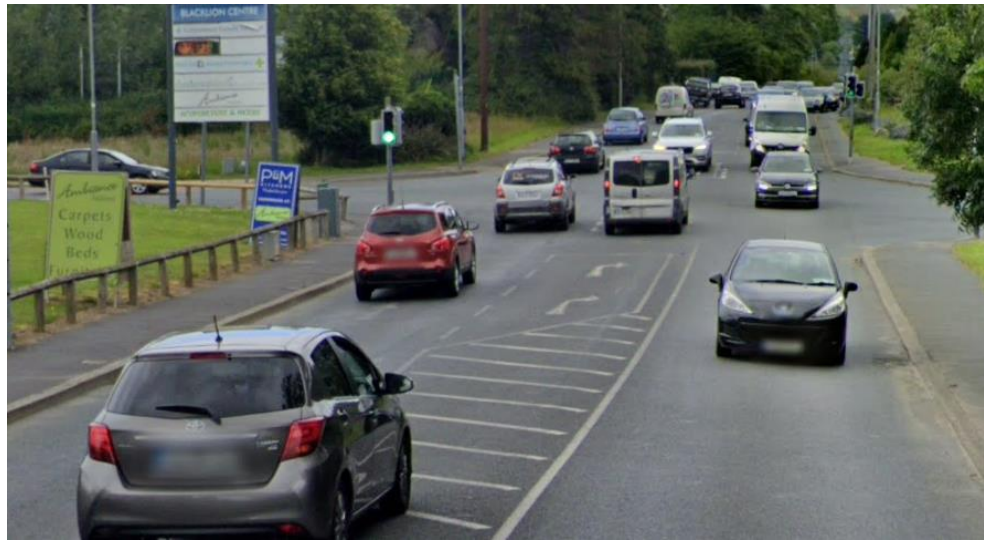
Figure 3-2: R761 Regional Road at the Redford Park Junction
