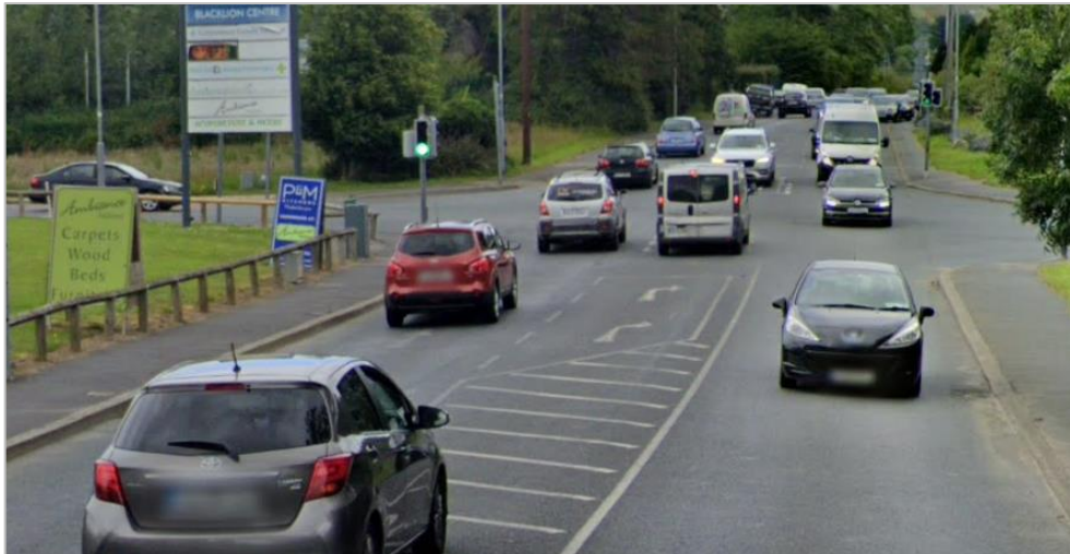
Figure 3-2: R761 Regional Road at the Redford Park Junction
